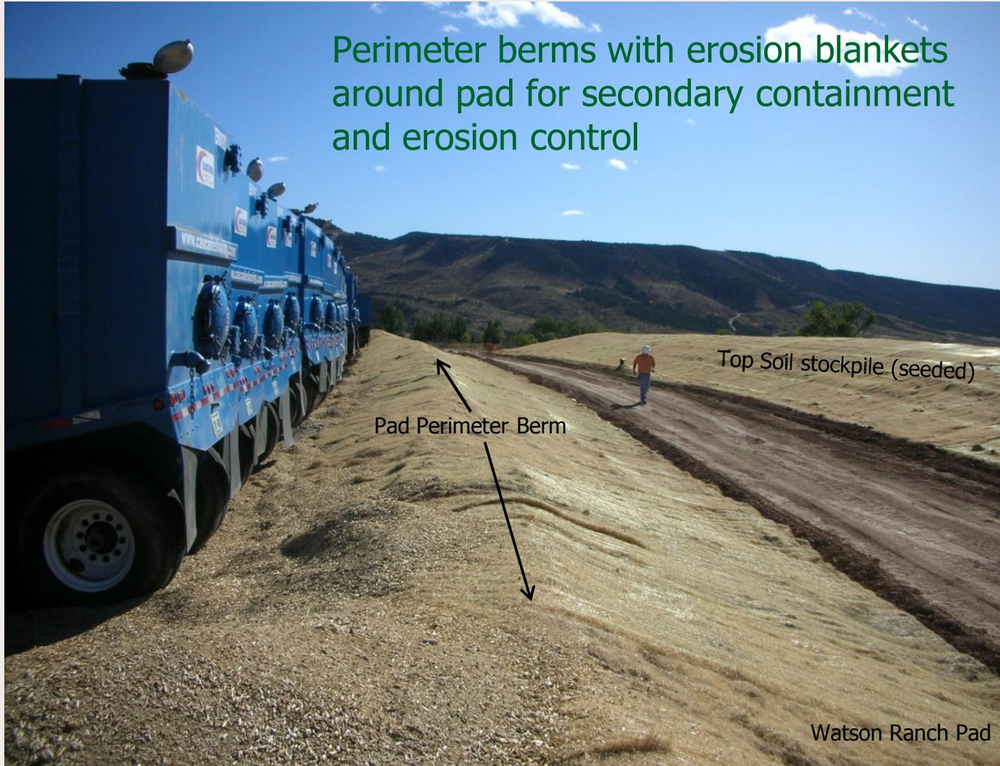
Perimeter berms with erosion blankets around pad for secondary containment and erosion control
