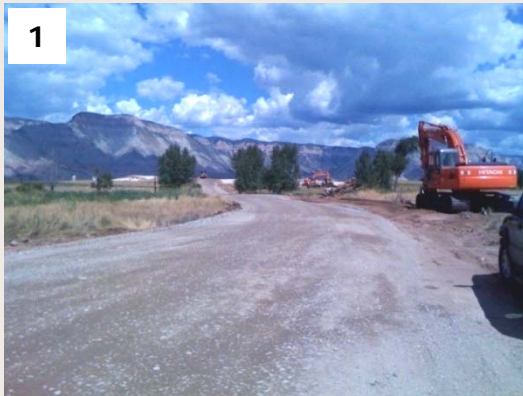
Access road is built
