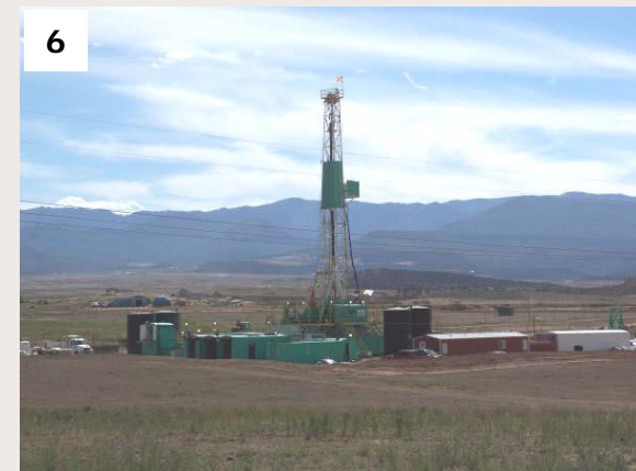
Drilling rig begins drilling surface hole and then production hole
