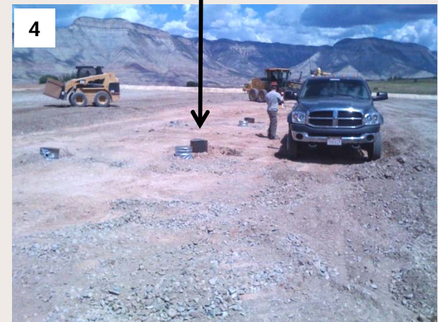
Conductors holes are drilled (cellars not yet installed)
