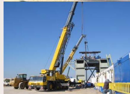
Drilling rig mobilizes and is assembled
